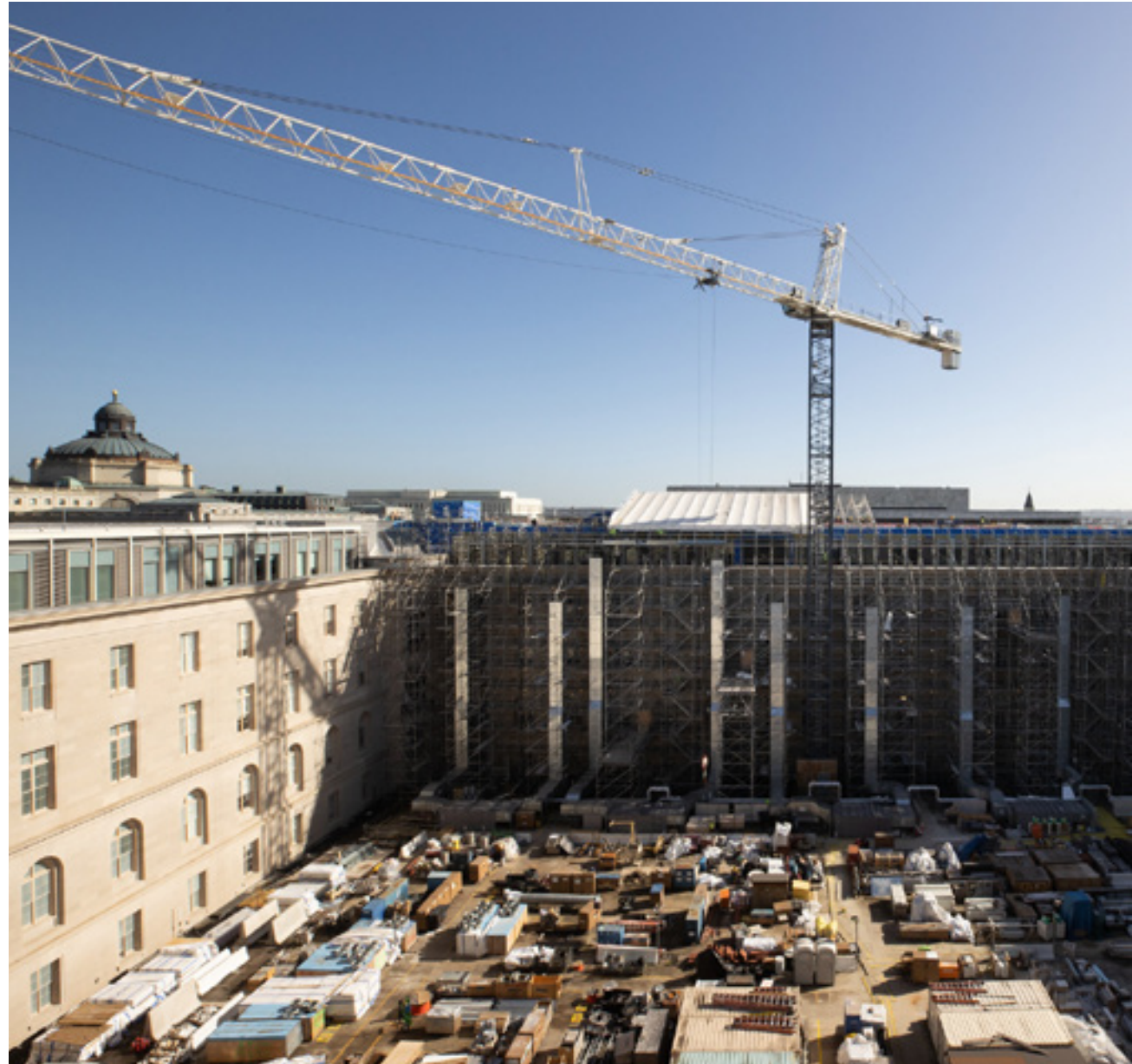
The Cannon House Office Building began a holistic renovation in 2014 which is approaching its final phase in 2025.
